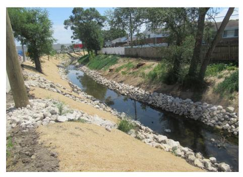
This Project included stabilization along 2,278 linear feet of eroded streambanks, installation of 2 natural rock riffle structures, vegetation management with 1.36 acres of native plantings along the creek. The project will substantially improve water quality along Silver Creek. Funding was provided by the Village of Melrose Park along with a grant from the Illinois EPA Section 319(h) Grant Program.
